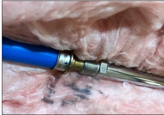
Figure 9.47 Insulated Hydrant to Prevent Freezing
