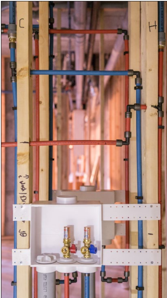
Figure 9.13 PEX tubing Installed in Wood Studs
