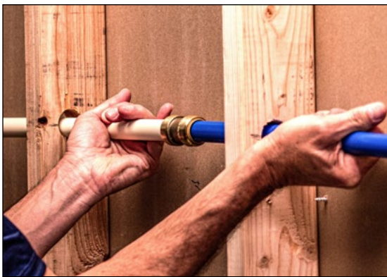
Figure 9.39 Push-Fit PEX Transition Fitting to CPVC
