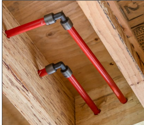
Figure 9.6 Elbow Fittings in a Confined Joist Cavity
