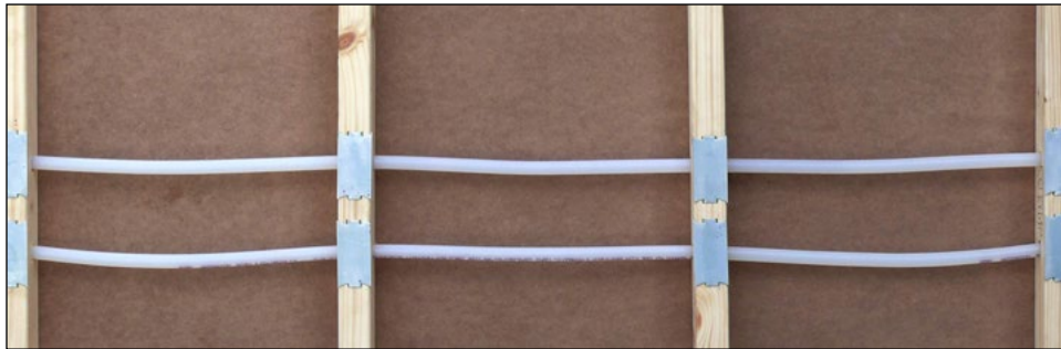
Figure 9.24 PEX Tubing Installed with 1/8 inch Slack Per Foot
