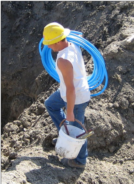
Figure 10.1 Worker Carrying PEX Tubing
