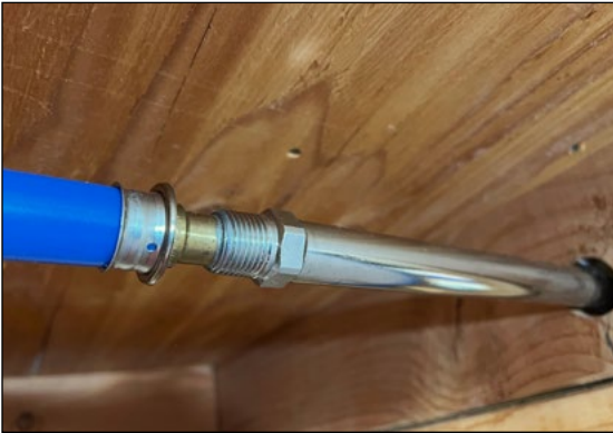
Figure 9.46 PEX Connected to a Hose Bibb/Wall Hydrant
