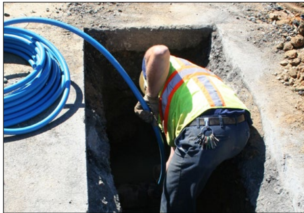
Figure 10.10 Installing PEX Tubing as an LSL Replacement
